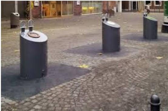
The design of underground bins varies considerable and in turn so can the collection methodology and impact on the street environment. The designs seen in the UK predominantly fall into three types: those relying on a hydraulic platform to house 'standard' bins, bottom opening crane lifted, and top opening crane lifted.
